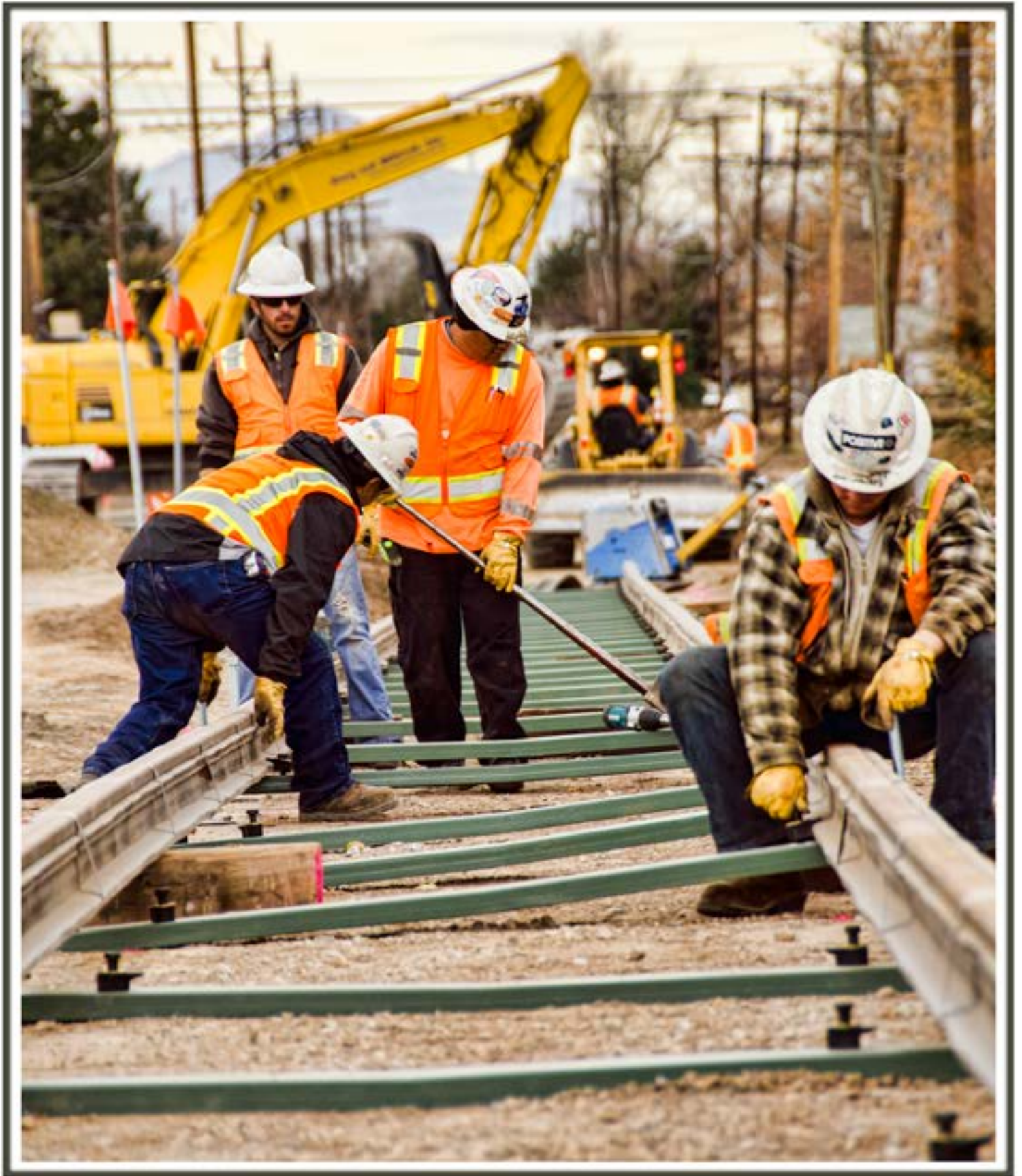
Stacy and Witbeck Inc, Suarhouse street car track crew, stabilizing the rails in preparation for a cement pour.
